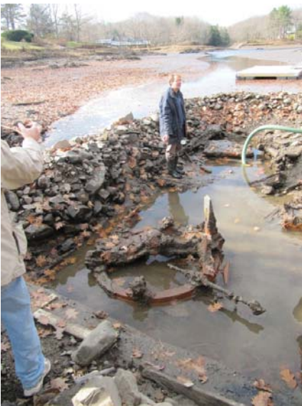
Low tide exposes the 19 th century turbine.
